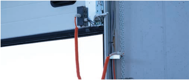
Cable break or spring break safety device
